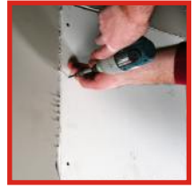
Gypsum board application
