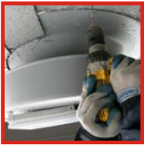
Fixing Air handling unit & Ventilators
