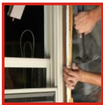
Doors & window framing
