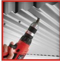
Cement Sheets Roofing
